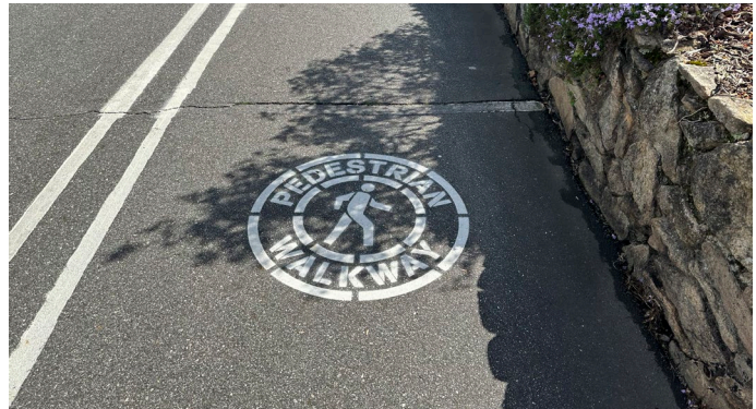
Pavement markings identify this area as a walking lane for pedestrians in the absence of a sidewalk. Physical protection should be provided with vertical separation in the striped buffer space.
