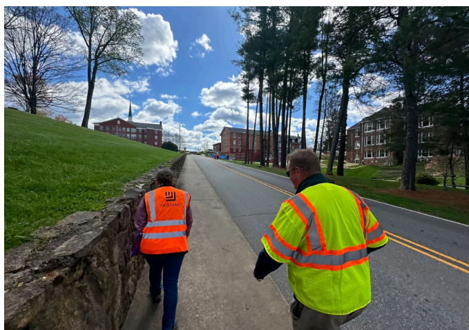
Bailey St is constrained near downtown and the MHU campus with a retaining wall and steep slopes.
