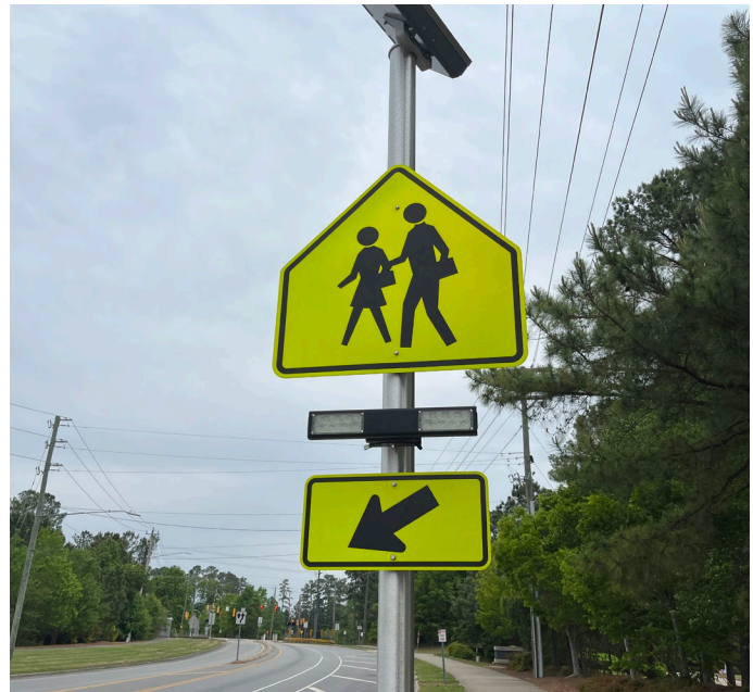
At either end of the midblock crossing, a signal should be installed that allows pedestrians to activate the flashing beacon.
