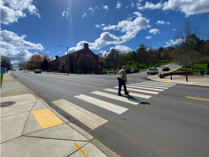
A pedestrian crosses Cascade St at Joe Anderson Dr, where existing travel lanes are as much as 18 ft wide.
