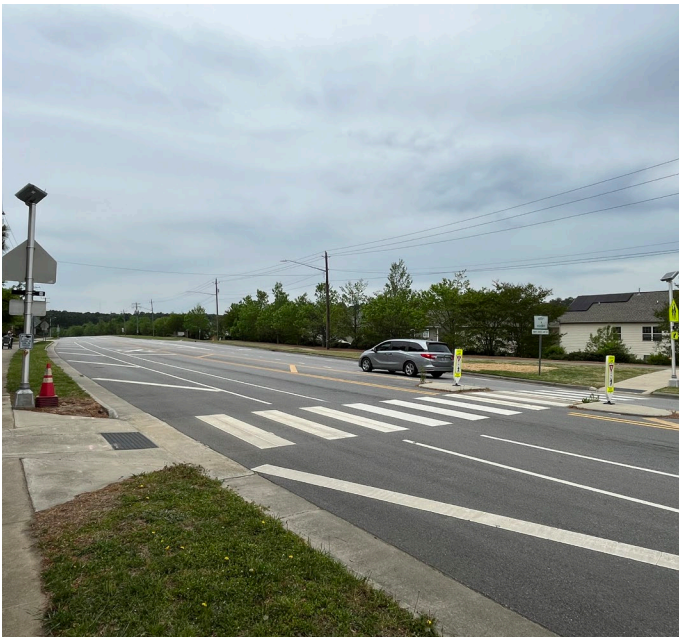
Midblock crossings, such as this on Laura Duncan Rd in Cary, NC, should feature high visibility crosswalk markings in addition to signage. A pedestrian refuge island may be provided if the roadway is wide.
