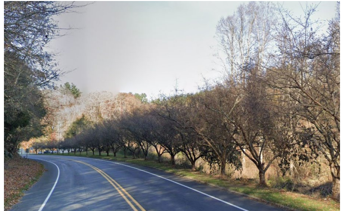
Existing trees may need to be removed and retaining wall installed where shoulder slopes down to Gabriel Creek.
