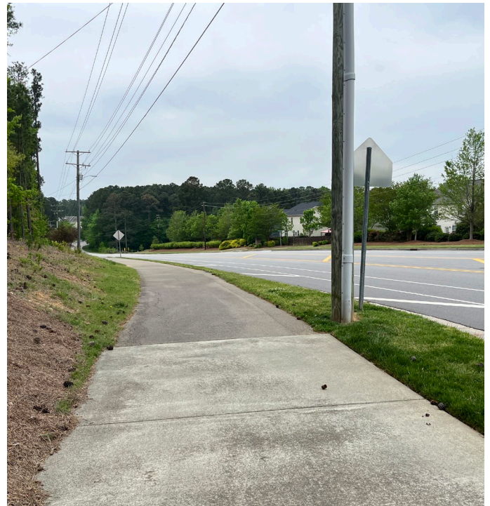
A concrete sidepath turns to asphalt at the border between Cary, NC and Apex, NC on Laura Duncan Rd.
