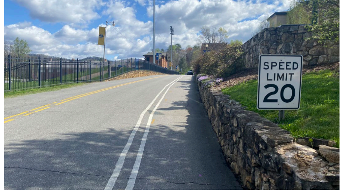
A pedestrian walkway was recently striped on the southern portion of the east side of Athletic St.
