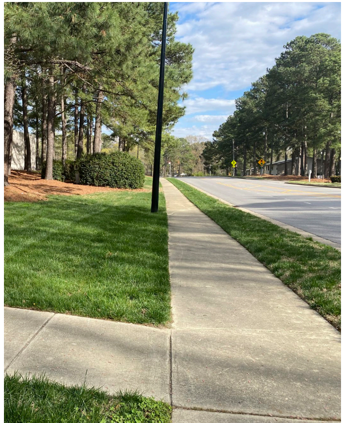
Sidewalk on 7th Ave in Garner, NC features a planting strip buffer
