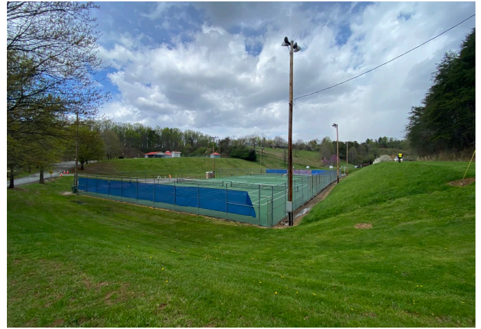
Slope conditions adjacent to the roadway present a challenge for developing bicycle and pedestrian facilities.
