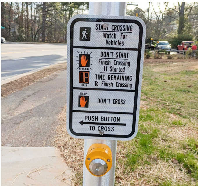
A push button is often provided to request a pedestrian crossing phase at an intersection. Credit: City of Raleigh
